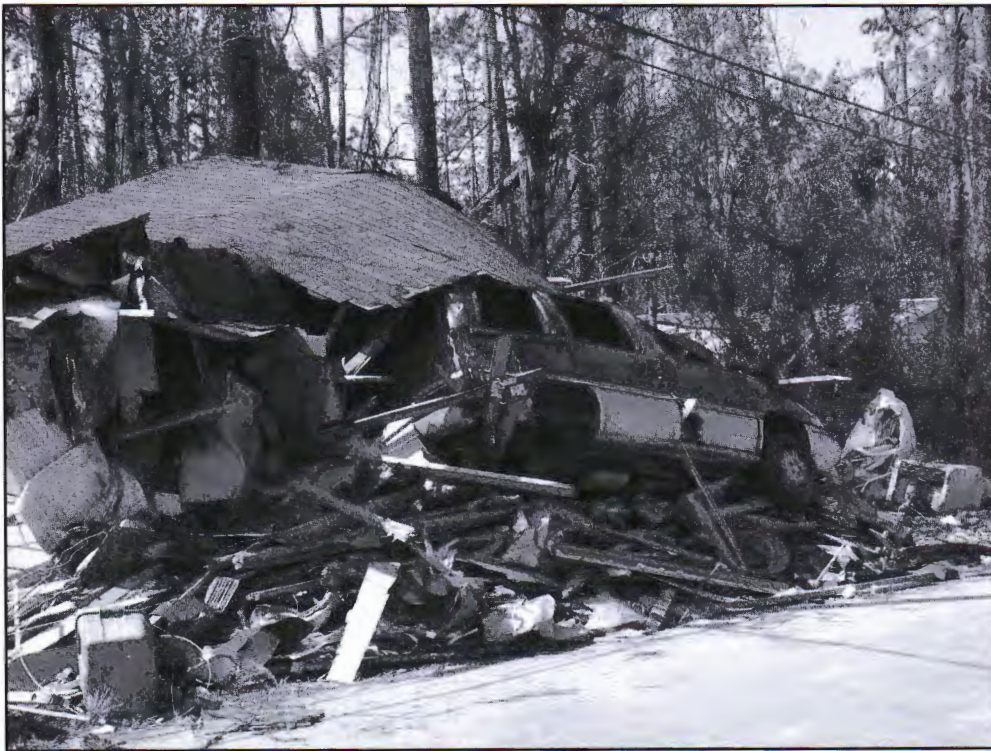
Waveland, MS - water pushed this van deep into the debris as it washed through and devastated the Waveland, MS area.
