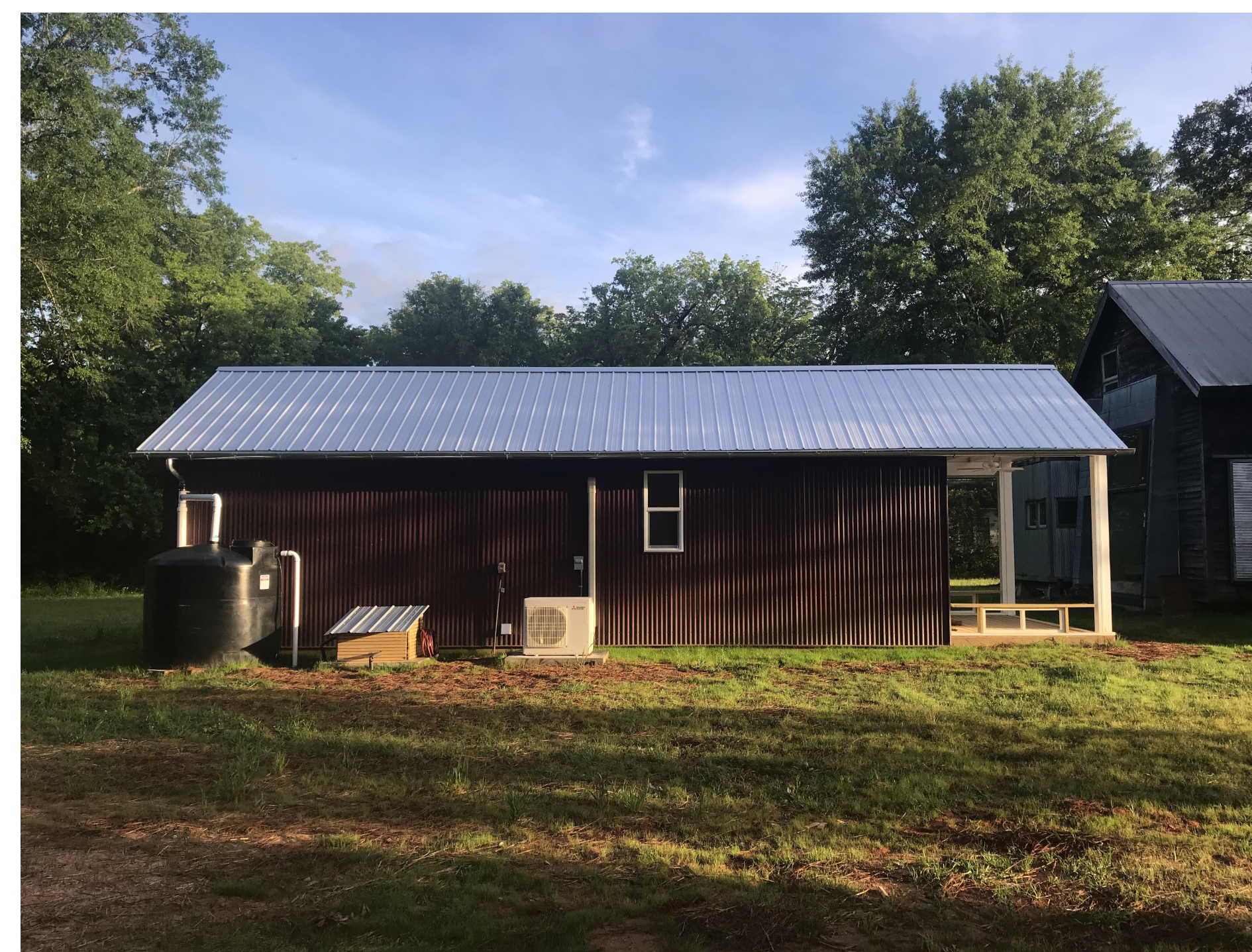
Figure 1 - Completed home with rainwater harvesting system installed.
