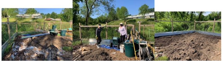
Painted 100 cement blocks for front wall, cleared and leveled ground, laid weed barrier, gravel, built and leveled block wall using dry stack method.
