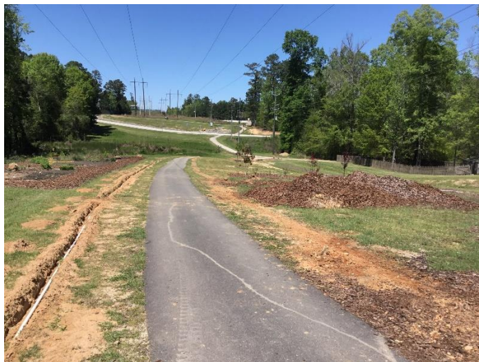
Installation of Irrigation and Multi-use Trail Extension
