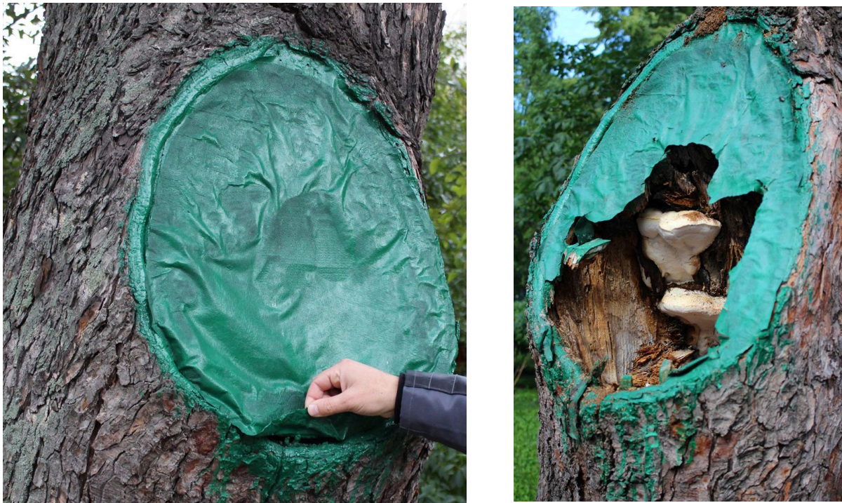
Figure 6a-b. Pruning paints did not prevent decay in this horse-chestnut ( Aesculus hippocastanum ) tree.
