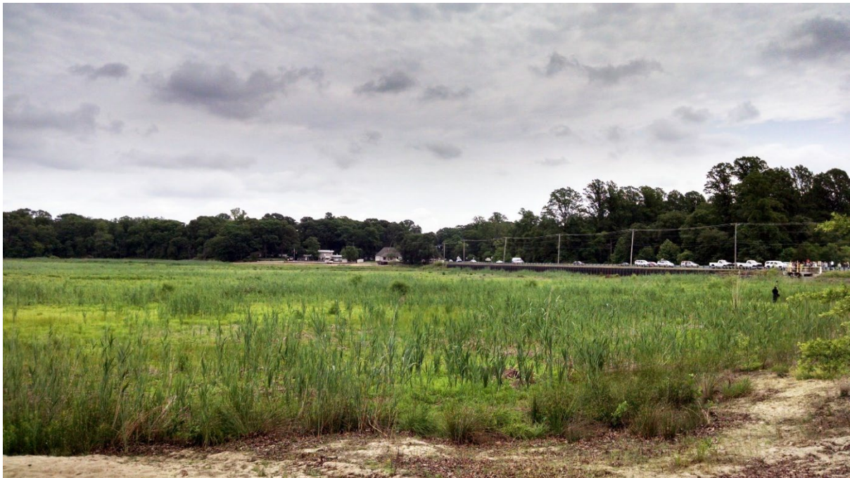
Figure 1. Sunset Lake in 2015 before the dam repair was completed. On the right of the photo is a human figure in black that gives a sense of scale of vegetative growth. (Photo credit: Sal Mangiafico.)
