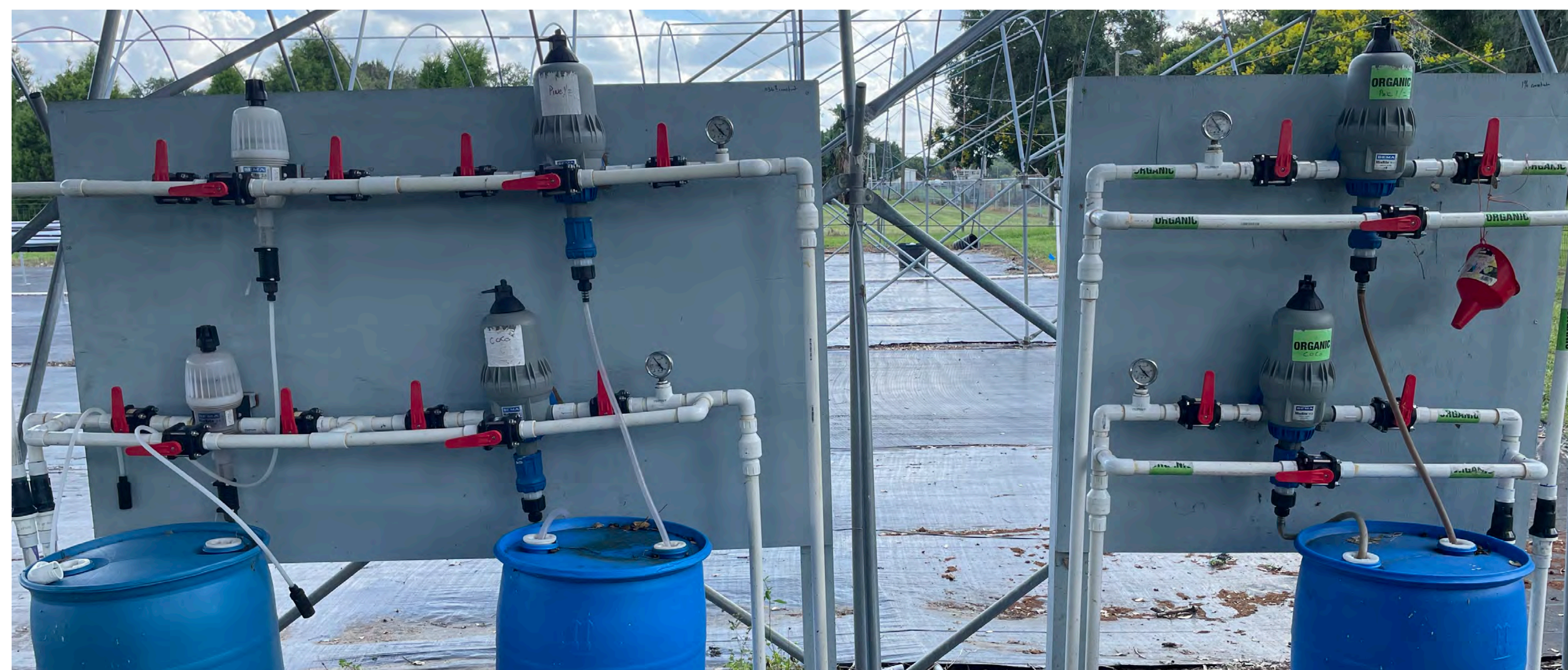
Figure 3: Fertigation dosatron injection systems. Left: two parallel systems for injecting NPK mixtures and calcium products separately. Right: injection system of the organic trial Multizone in each setup to allow for changing fertigation needs for different substrates.
