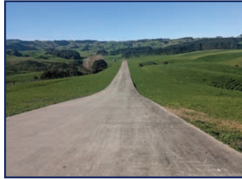
All Weather Runway: New Zealand producers are very focused on timely fertilizer applications on perennial ryegrass. This runway allows access for planes to load fertilizer and make aerial applications on the steep terrain, regardless of wet conditions.
